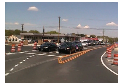
Construction at the base of the bridge
