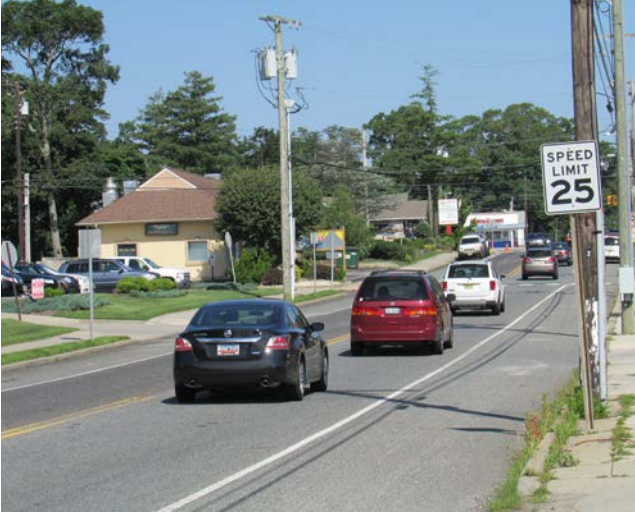
Poor sidewalk maintenance on Maryland Avenue near Shore Road, facing west
