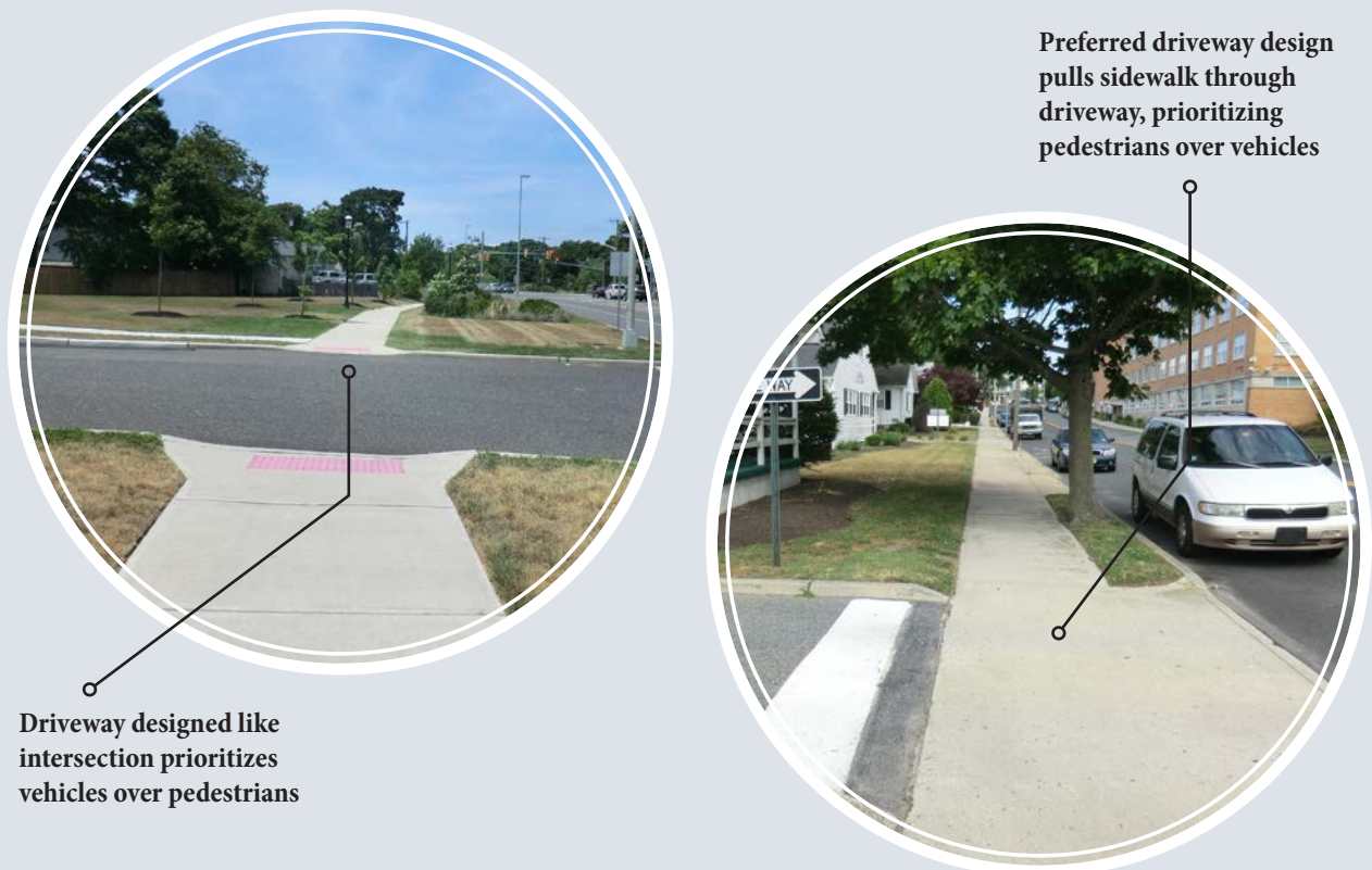
Figure 8-4 | Example Driveway Designs in Somers Point
