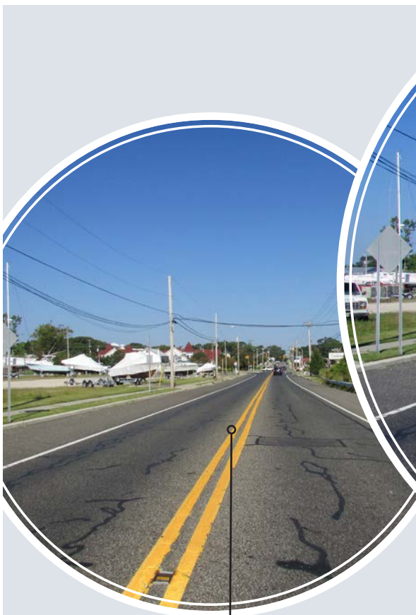
Figure 8-40 | Maryland Avenue Existing Alignment
