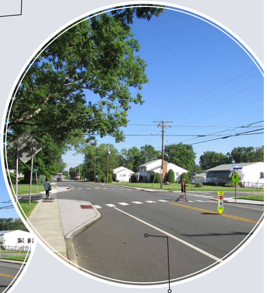
Figure 8-23 | West Laurel Drive Photosimulation Simulation showing curb extensions to shorten crossing of West Laurel Drive and calm traffic, as well as improved signage
