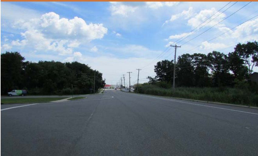
Roadway widens near intersection with NJ Route 52 (facing east)
