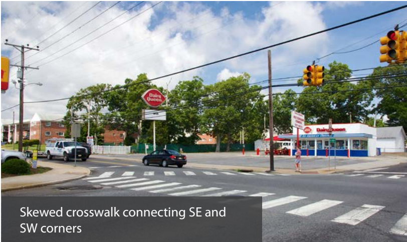
Continental crosswalk striping but no pedestrian signal heads, facing south
