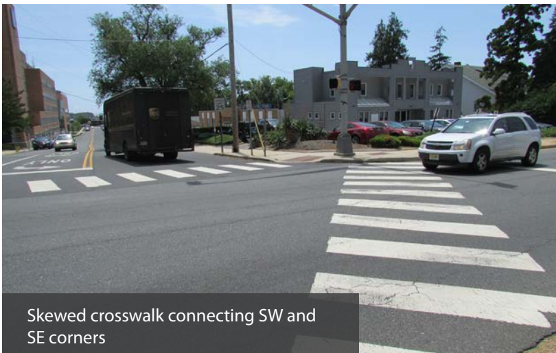
Eastbound and westbound approaches of New York Avenue are offset, making circulation for all modes more difficult
