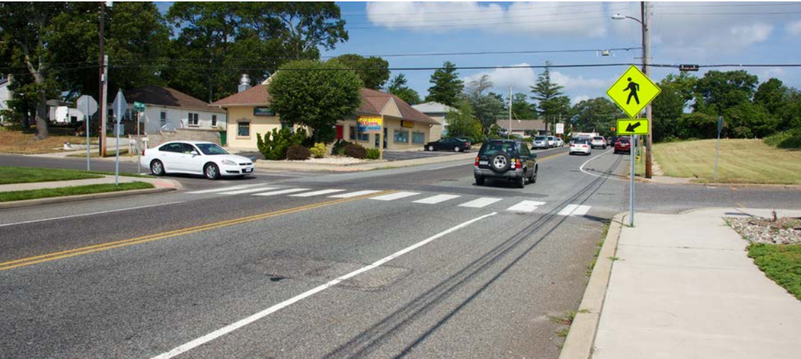
Continental crosswalk striping and signage improve the visibility of the crossing of Maryland Avenue at Sunny Avenue (Maryland Avenue, facing west) (Maryland Avenue, facing west)
