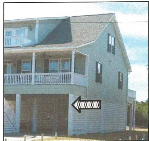
F2.c6: Latticework screen hiding most of pilings
