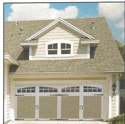
G2.d: Garage doors relate to house style and dormer features. Design creates a pedestrian scale
