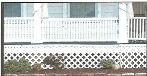
Continuous latticework ignores rhythm of porch columns
