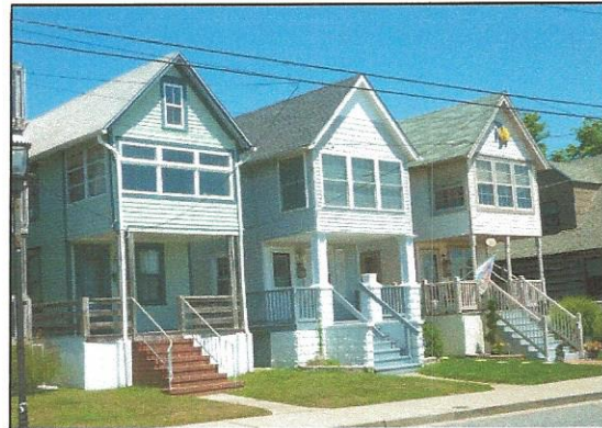
The foundation, especially when exposed as many are in the Historic District, is important to the character and feel of the house.
