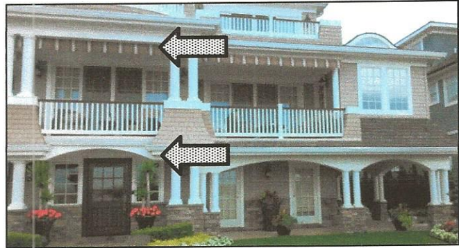
F2.b: 'False' first story imitates vertical elements of higher levels
