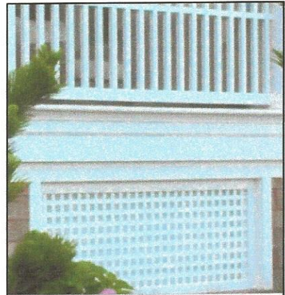
G2.c: False panel duplicates scale and pattern of elevated porch rail
