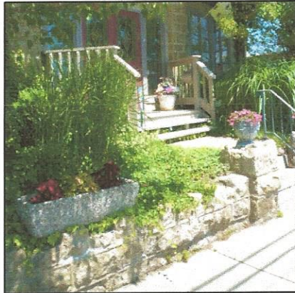
Retaining wall for small setback
