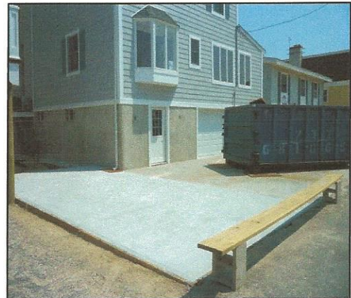
E2.c.1: Inappropriate type and excessive paving
