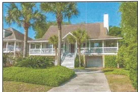
H2.b1: New house in Charleston synchronizes in setback, porch detail and landscaping with historic suburban neighborhood
