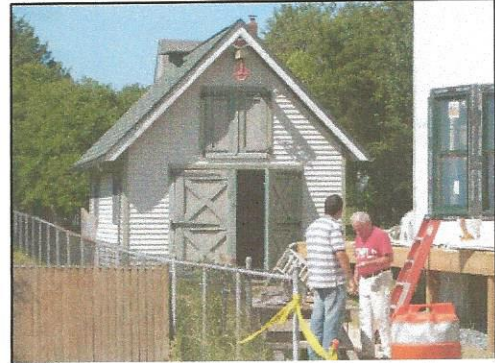
E2.f.2: Contributing garage retained during demolition of 1910 house
